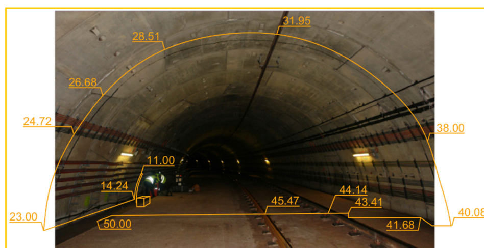
Figure 66. Monitored tunnel section [150].
