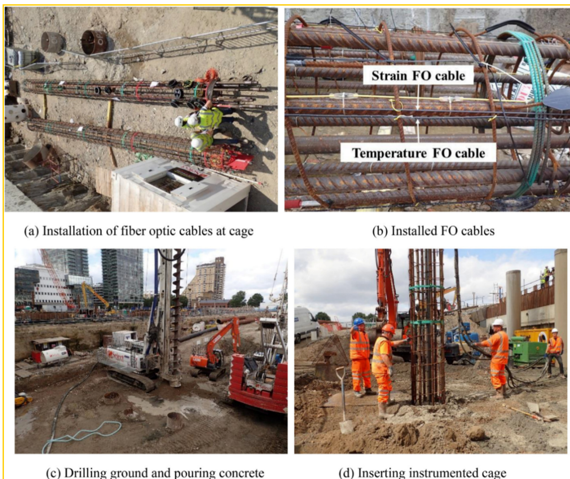
Figure 50. Installation of the DOFS and the pile [7].
